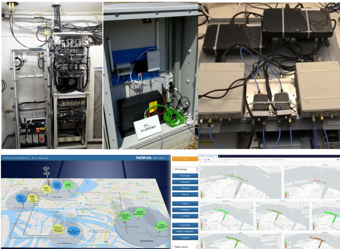
Figure 7: Hamburg Smart Sea Port testbed: base station at Hamburg TV tower (upper left), device installation for traffic light (upper middle), multi-connectivity device as installed on barges (upper right), slice lifecycle mgmt. tool (bottom left), KPI panel (bottom right)
