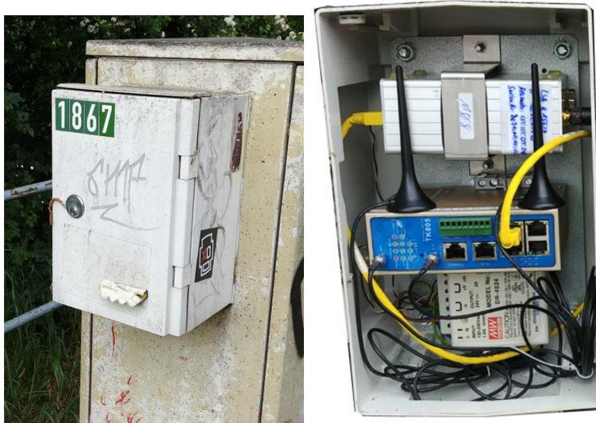
*Figure 5-6: Hardware and containment for traffic light integration*
