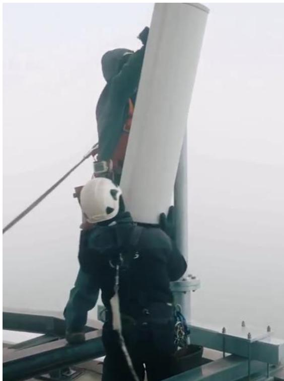
*Figure 7-30: Mounting of the antennas of the base station*
